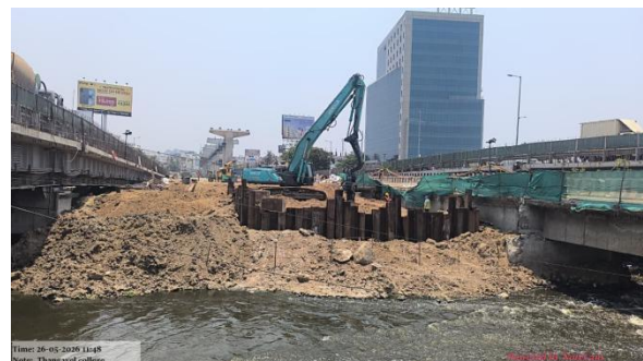
Fig 10 — Wide-angle view showing scale of earthwork inside the waterway.
