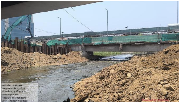
Fig 7 View from beneath existing road bridge: flow cross-section reduced to 7.89 metres (Google Earth / Airbus, 26 April 2026).
