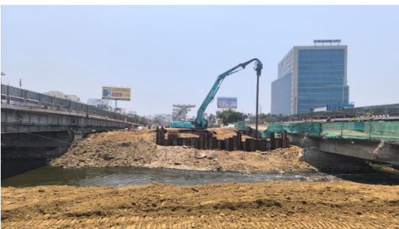
Fig 9 — Under-bridge view and work carried inside the Okkiyam Maduvu
