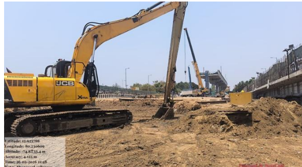
Fig 8 Construction works inside Okkiyam Maduvu; pre-construction channel width significantly constricted.
