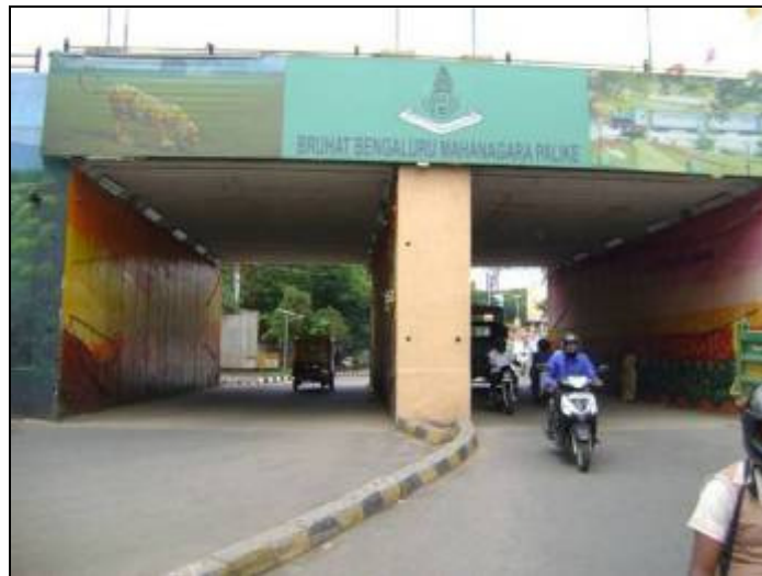
Plate 4-7 View of At-grade Road below Grade Separator at Palace Road Junction
