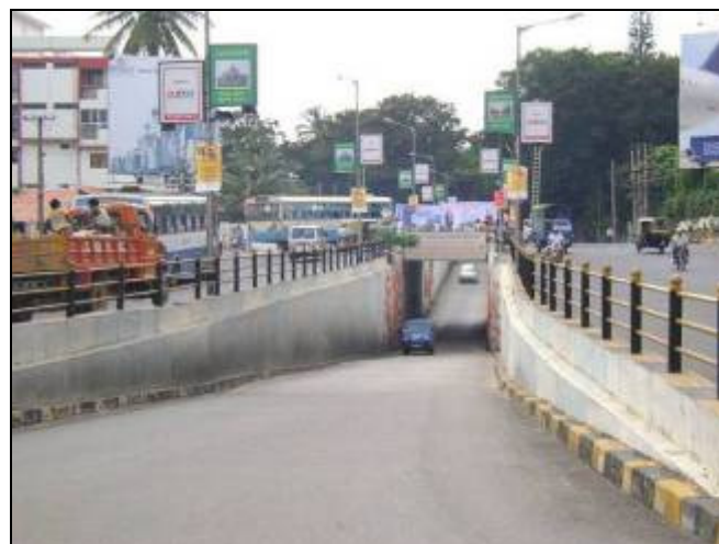
Plate 4-10 View of Underpass at Cauvery Theatre Junction
