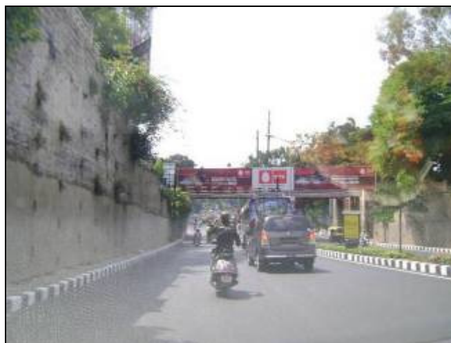
Plate 4-6 RUB Near Kumarakrupa Road Junction
