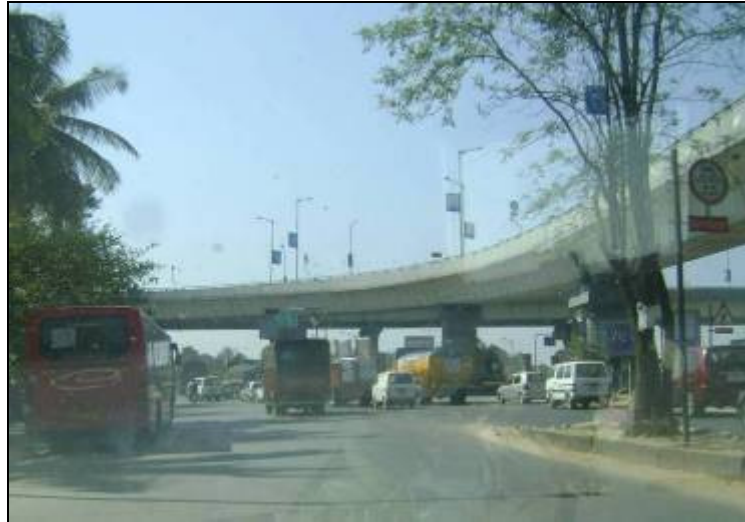
Plate 4-18 View of at-grade road at Hebbal Junction
