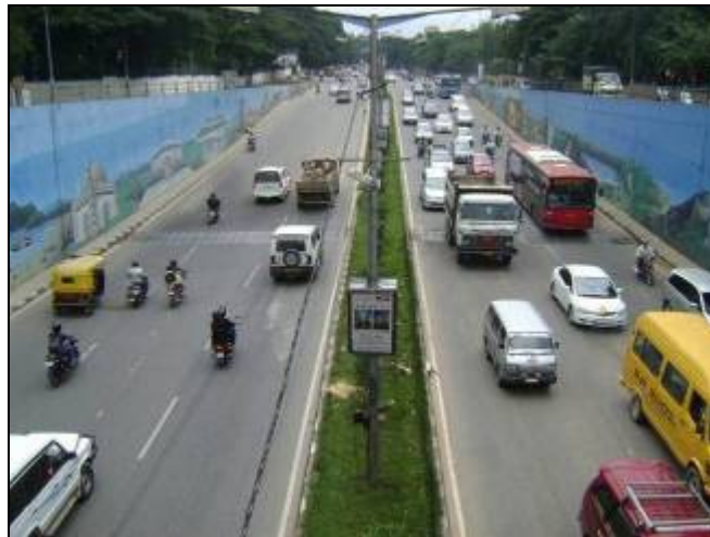
Plate 4-11 Existing underpass at Mekhri Circle along NH-7
