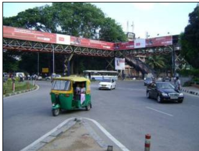
Plate 4-3 Pedestrian Skywalk at High Grounds Junction
