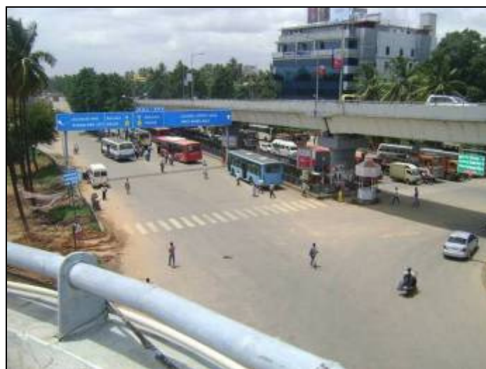
Plate 4-20 Aerial view of ORR towards kolar at Hebbal Junction
