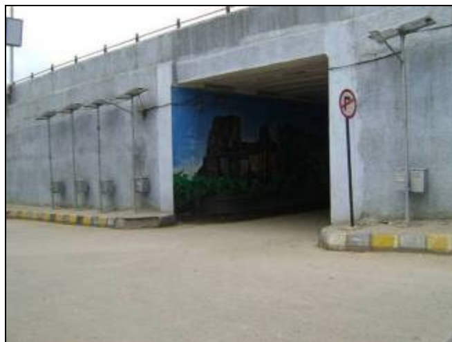
Plate 4-16 View of vehicular underpass at CBI Junction
