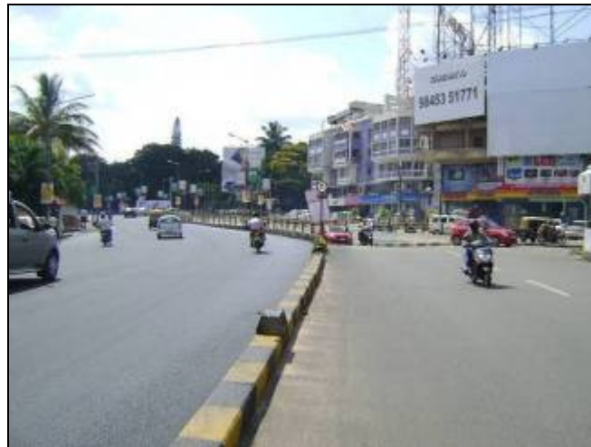
Plate 4-9 View of Sanky Road Up-ramp at Cauvery Theatre Junction
