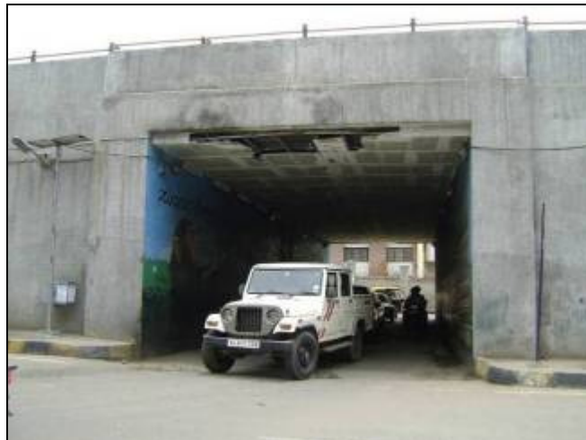
Plate 4-14 View of vehicular underpass at Sanjaynagar Road Junction
