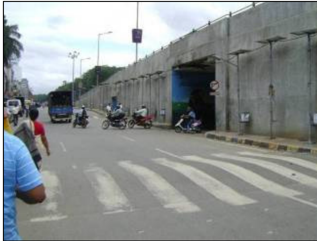
Plate 4-13 View of at-grade service road
